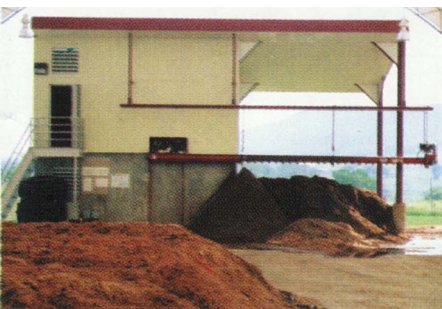
Separator House With Stacking Auger And Covered Composting Pad.
