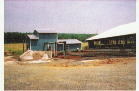
Housing For Sand & Solids Separation With Horizontal Auger & Stacking Pad.
