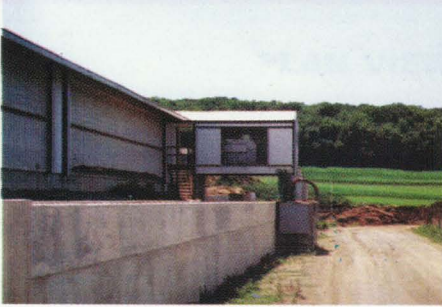
Above Ground Reception With Drive-Under Separator Building.
