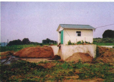
Separator House Directly Over Reception Pit With Stacking Pad.
