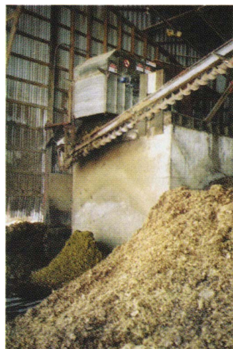
Separator & Solids Management In Former Commodity Shed.
