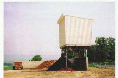
Park-Under Separator And Solids Management Pad.
