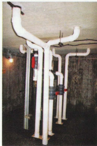
Mechanical Space Between Separator (Above) & Reception Pit (Below).
