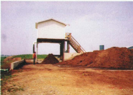
Drive-Under Separator Building With Solids Management Pad.
